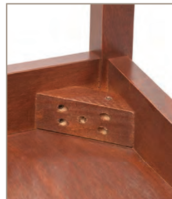
Corner block strengthens corners
